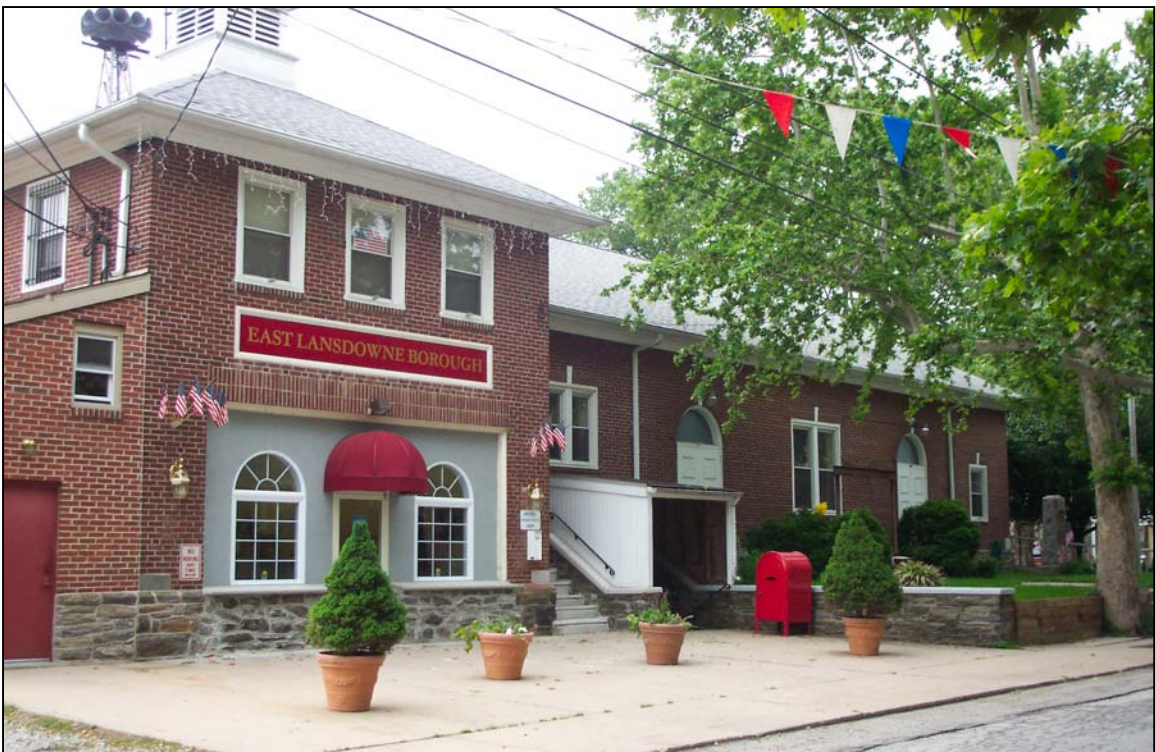
East Lansdowne Municipal Building
